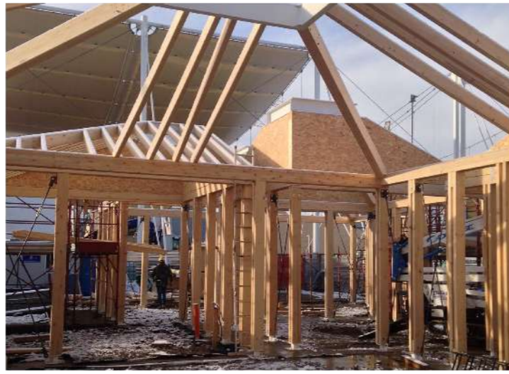
2. The wooden structural frame
