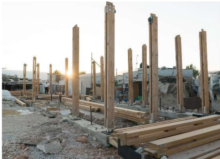
4. The vertical wooden posts of the structure
