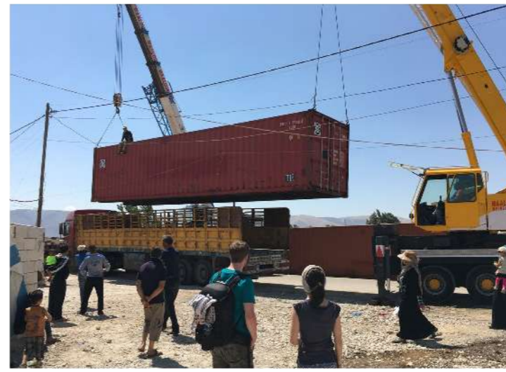
3. A shipping container being used as a building component
