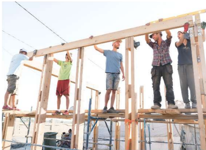
5. Workers constructing the roof structure
